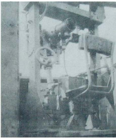
*Uhu operator's chair and viewer, the elevation control is on the left side*
